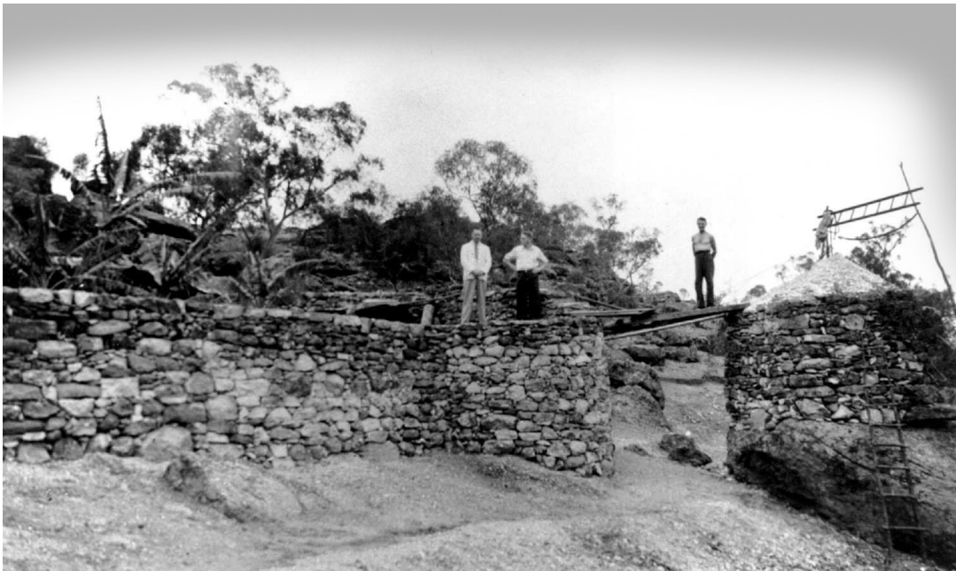
An elaborate series of retaining walls, terraced gardens and cisterns were constructed by Valerio, working alone and at night for his hill hideaway. (Image credit: Griffith City Council)
